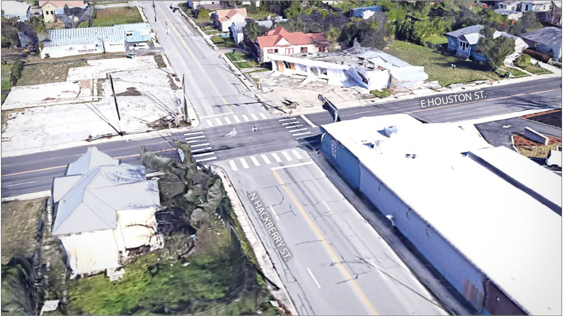
Figure 11: Focus Area #1 Transformative Project – Houston Street and Hackberry Street (Existing)
